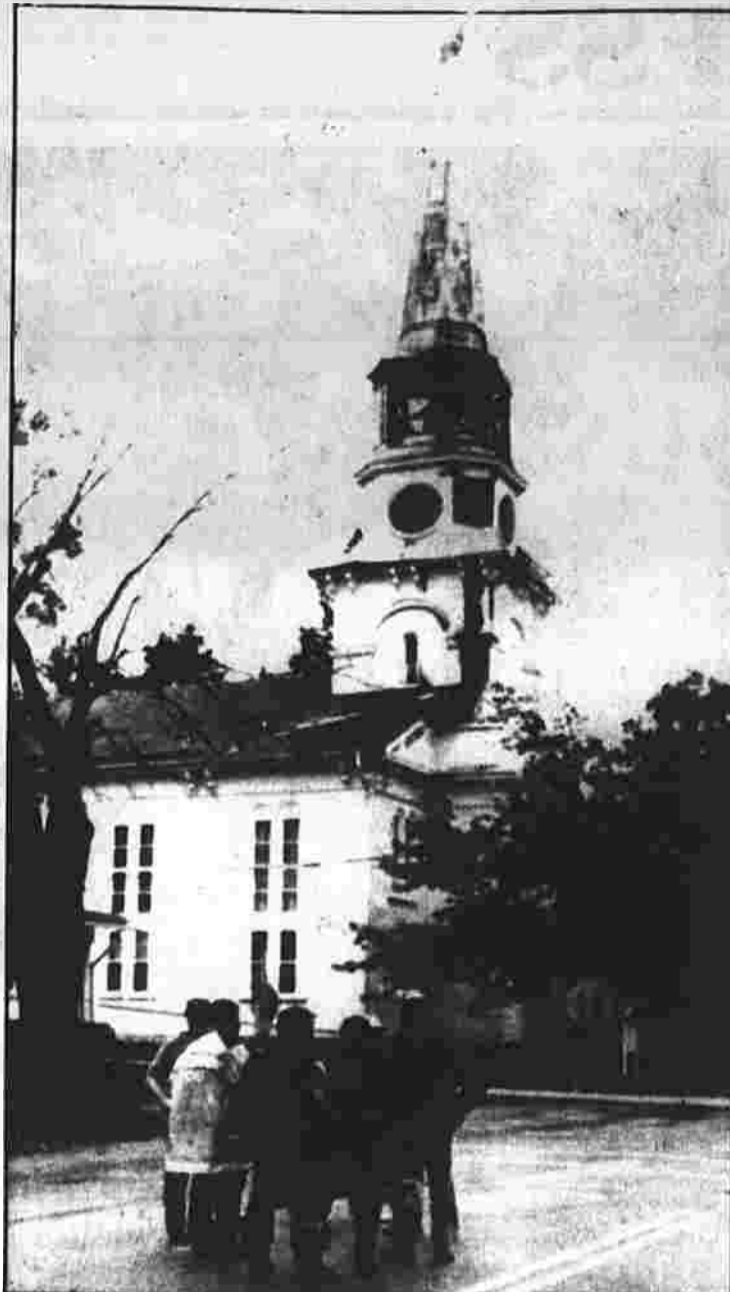
Church fire: Firefighters and residents stand near the 130-year-old Thompson Congregational Church, the steeple and roof of which were badly damaged by a fire Monday morning. Firefighters from nine communities battled the blaze at the church at Routes 193 and 200 for about five hours before bringing it under control. Officials believe the cause of the fire was electrical.
